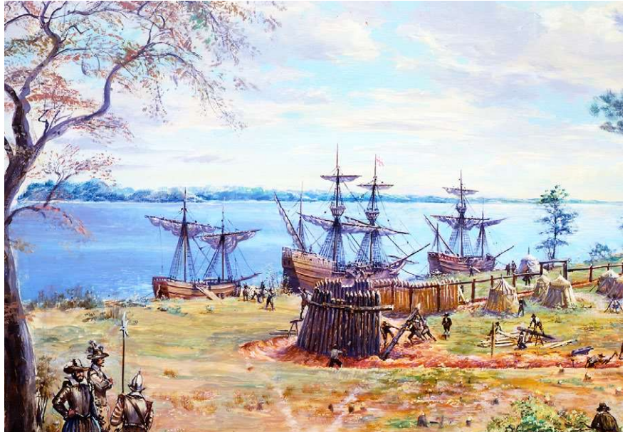
Painting depicting the James Fort construction in May-June 1607.
